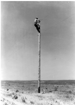
Figure 3. An REA lineman at work on the Great Plains.
